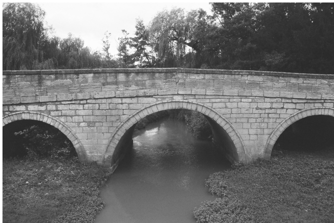
The 18 th century bridge over the Cock Beck in Aberford; the original width of the river is evidenced by two arches that are no longer used
